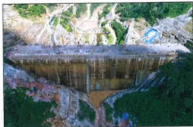
Curing of the upstream face.
