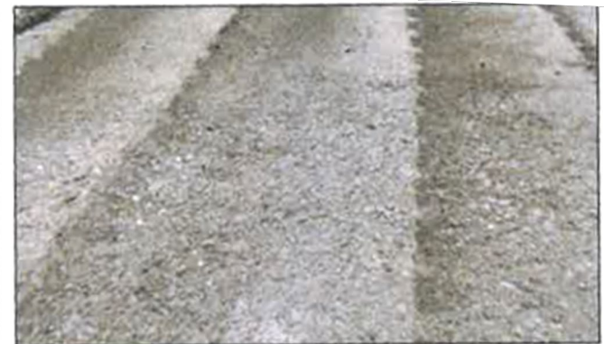
Cold joint treatment, showing the RCC surface after the steel brush treatment.
