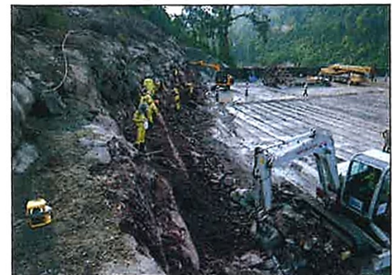
Rock foundation excavation and treatment.
